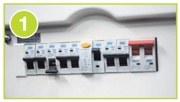
Before starting any electrical work, make sure that the mains supply is turned off at the consumer unit.
