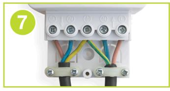
Fully tighten the terminal screws and make sure that no bare copper is exposed outside of the terminal.
