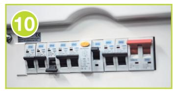
Restore the power to the circuit at the consumer unit and test.
