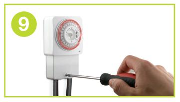
Refit the cover onto the front of the timer unit.
