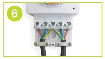
Insert the bare ends of the cable into the terminals as per the wiring instructions.
